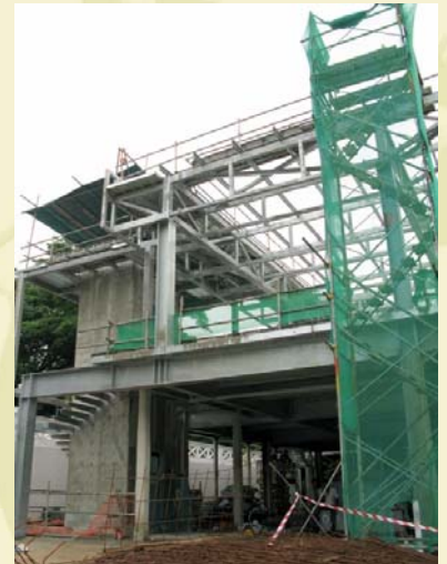
Glass Block Steel Structure Completed
